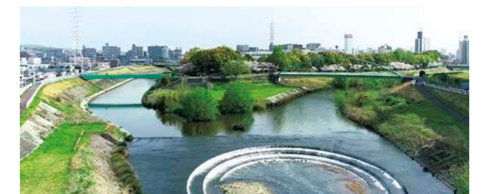
天白川と桶田川の合流点にある慶栄工 Construction designed for bed protection at the confluence of the Tempaku River and the Ueda River.
